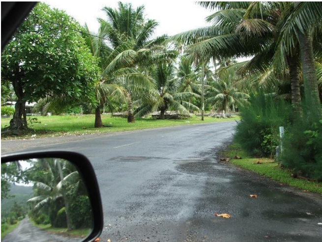
Un-prune hedges pose as a hazard to oncoming traffic.
