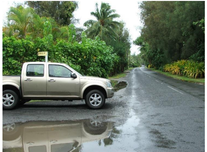
Safety hazard to vehicles connecting to main road.
